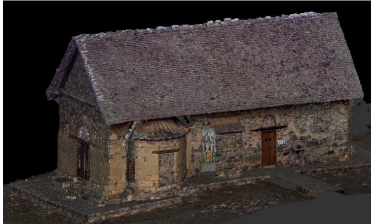
Figure 13: The merged point clouds after the cleaning procedure – work accomplished on site.
