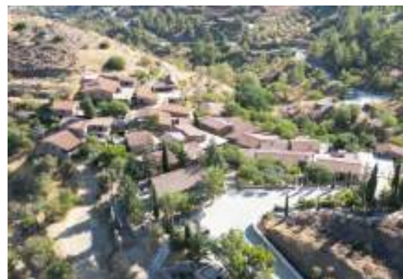
Figure 7: Drone Image, Southwestern entrance of the village.
