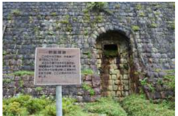
Figure 2. The Tonaru district of the Besshi Copper Mines is home to the remains of the ore sorting yard and the ore storehouse, as well as the aerial cableway for transporting ore and household supplies.
