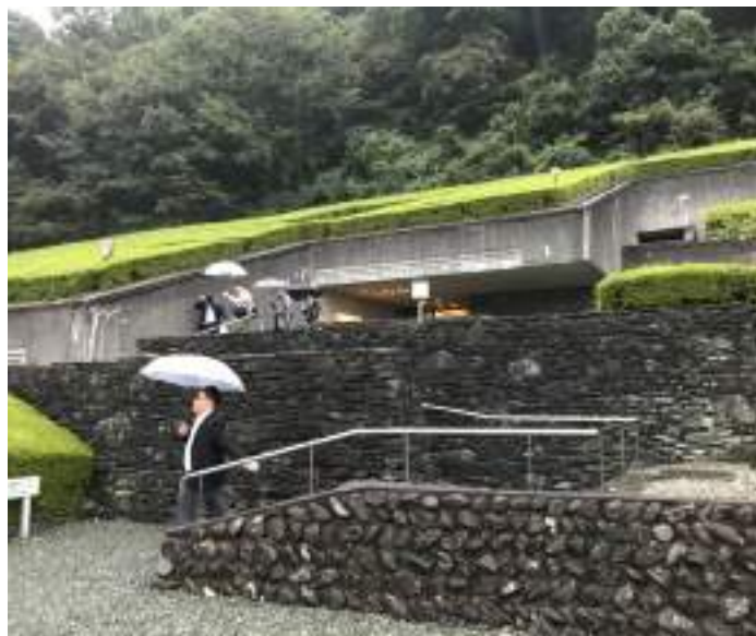
Figure 1. Besshi Copper Mine Memorial Museum's semi-underground building design resembles the underground mining tunnels. The interior is divided into five exhibition areas: Izumiya (Sumitomo's history), History, Geology (ore deposit), Daily Life and Customs, and Mining Techniques.
