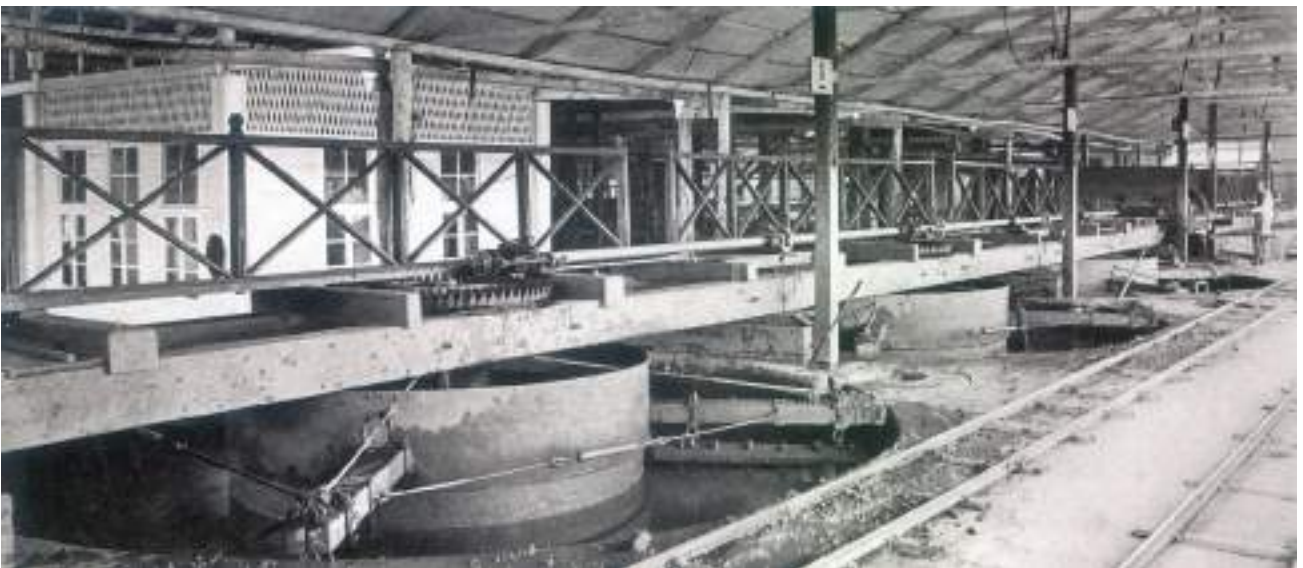
Figure 5. The giant mixer in the tin processing plant at Tambun, near Ipoh. (Photo credit: Leiden University Libraries Digital Collections)
