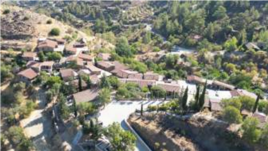
Fig. 4. Drone Image, overview of the Fikardou village
